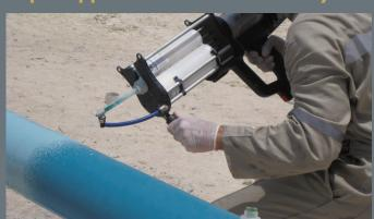
This rapid pneumatic spray system can apply Canusa's HBE liquid epoxy significantly faster and with less applicator error than standard brush-applied methods. The HBE Atomizer system setup includes:
