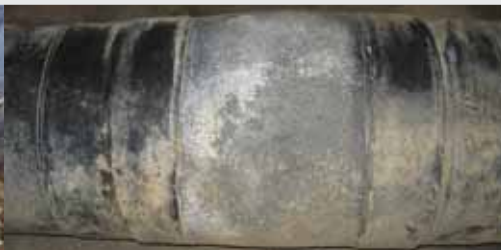
Over 15 years of in service sealing
