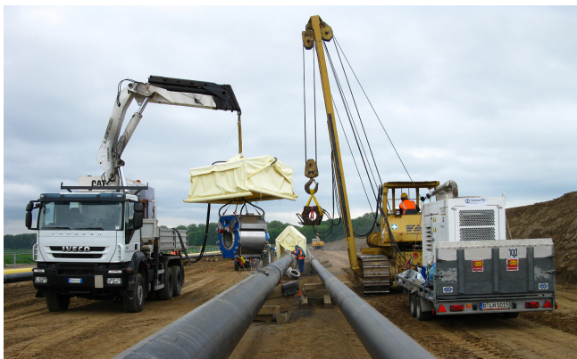
Figure 3. IntelliCOAT system used for onshore pipeline coating.
