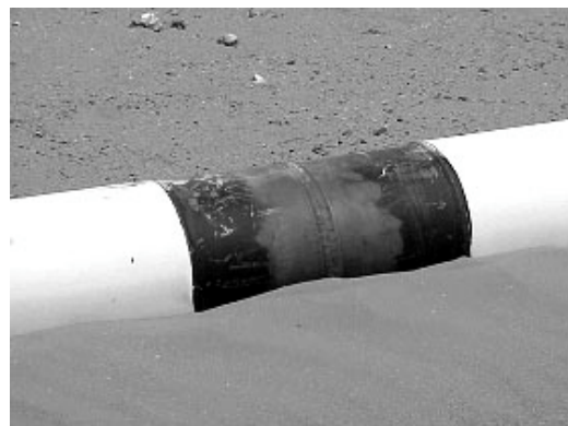
Partially Buried Cutback
