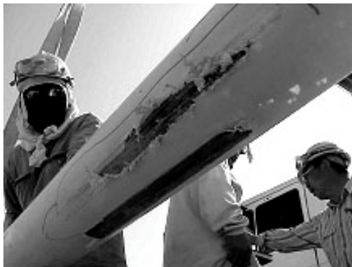
Coating Damage due to Movement
