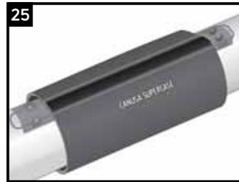
Measure a piece of CLR-200 closure material - 5 mm shorter than the full width of the CSC-XP-R and prepare the ends by cutting the corners off (1 by 1 cm) to reduce possibility of lifting. The CLR-200 is installed along the entire weld seam to prevent overheating during the application process.
