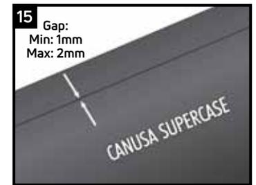
Gap between both ends should be adjusted to min. 1mm and max. 2mm prior to closing the clamp.
