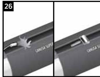
Ensure that the CLR-200 closure is fully conforming around the weld seam by rolling the full surface.
