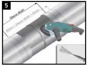
Ensure that the pipe is dry before cleaning. Using a power wire brush, abrade the pipe to a minimum of St3/SP3 (abrasive blast to Sa2.5/SP10 recommended). Lightly abrade the pipe coating adjacent to the cutback area to a distance of 50mm (2") beyond each end of the sleeve width using grit 40 - 60 sandpaper or P36 sanding disc.
