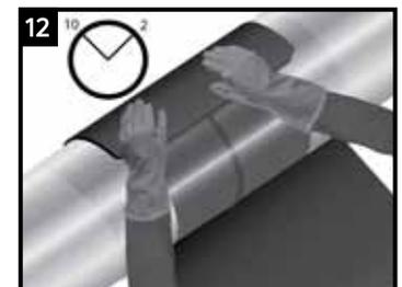
Place the underlap of the sleeve onto the joint, centering the sleeve such that the sleeve overlap is positioned at either the 10 or 2 o'clock position. Press the underlap firmly into place and use a roller to work out any trapped air. Feed the remaining length of sleeve under the pipe.
