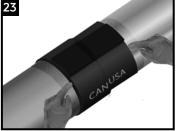
As a final check, ensure that the sleeve follows the entire contour of the surface and that there are no cold spots or burning of the sleeve. Make sure the edges of the sleeve are on tifting anywhere around the circumference of the pipe. This can be checked by feeling the edges all around the circumference of the steeve. If there is edge lifting, the edge should be reworked with additional heat.
